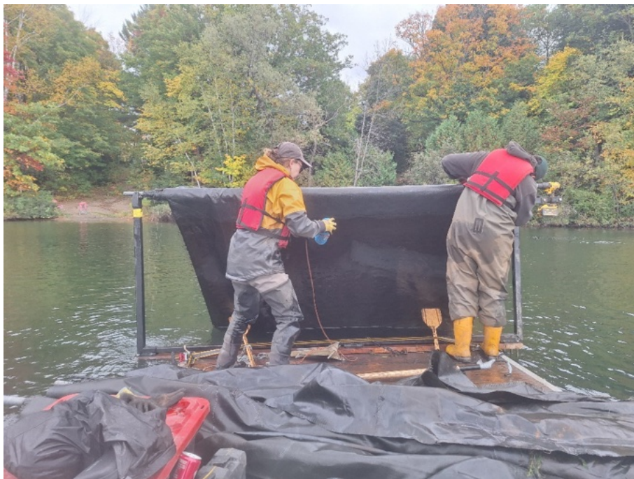
Figure11 : Removal of synthetic tarps.
