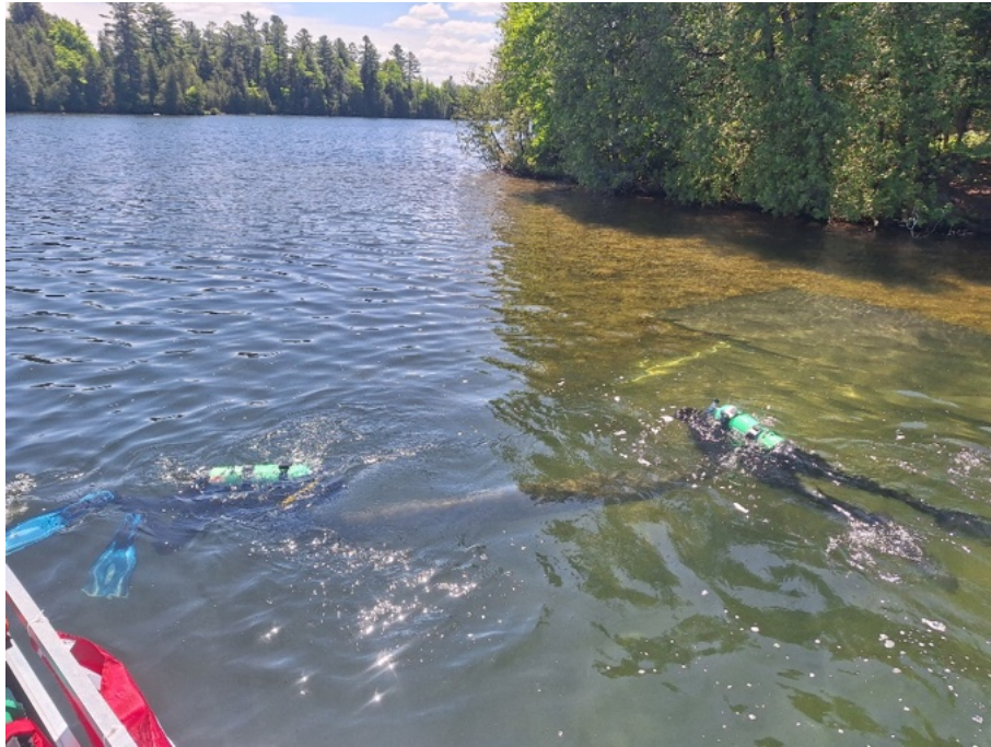
Figure10 : Installation of a synthetic tarp by two divers.
